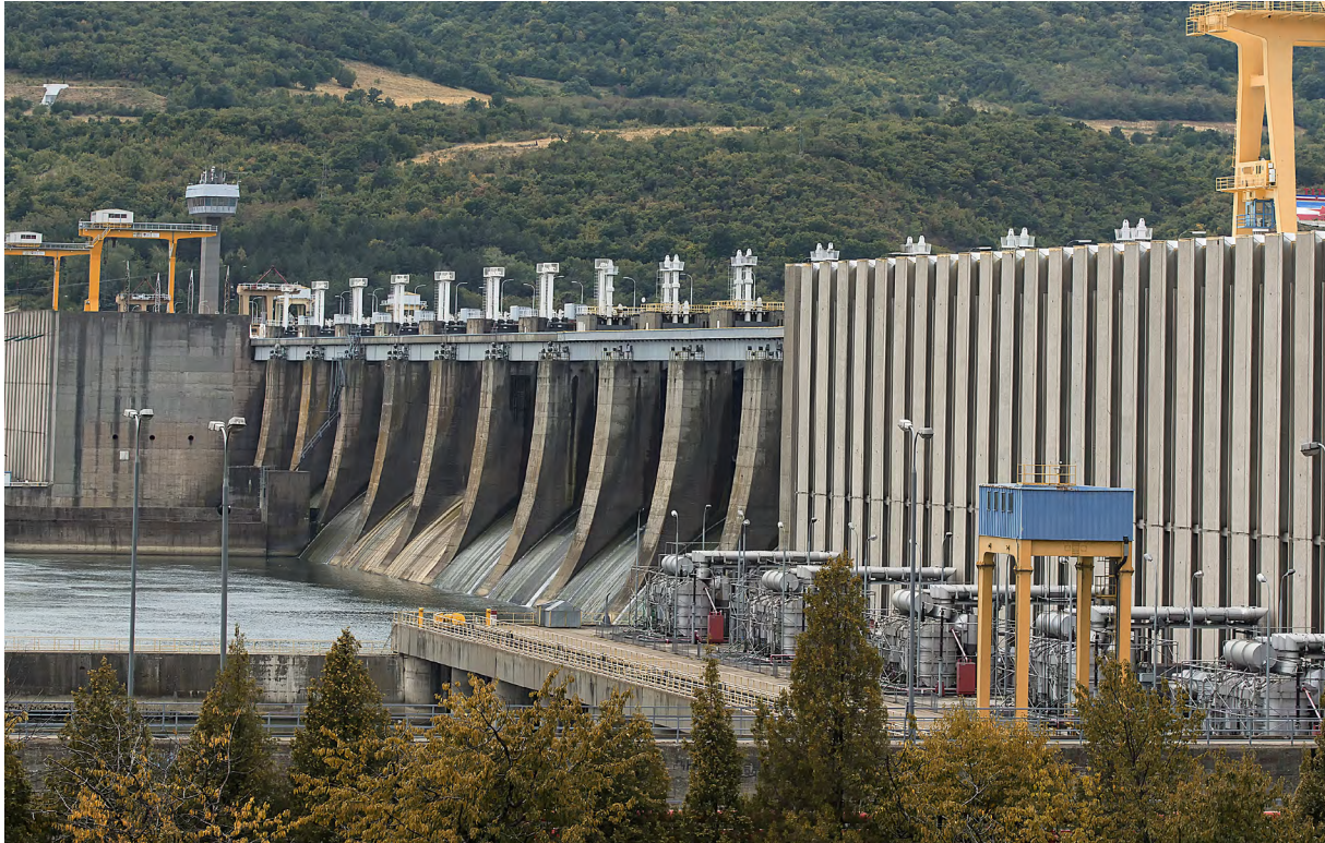
Fig. 11 Iron Gates I Dam, located at km 943 of the Danube River. Its construction changed the flowing regime of Danube upstream, from river to lake-like. This lake-like regime is evident up to Belgrade (Serbia)
